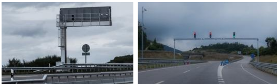
Figure 5 – Variable Message Signs and traffic lights. A-8 Motorway. Alto del Fiuoco (Lugo). Spain
