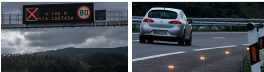
Figure 4 – Variable Message Signs and pavement beacons. A-8 Motorway. Alto del Fiuoco (Lugo). Spain
